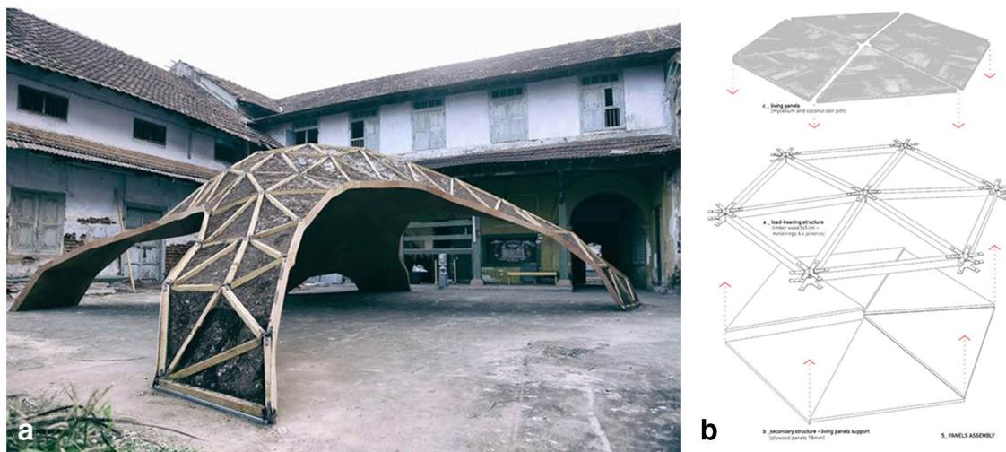
**Fig. 3** a Exterior Perspective of the pavilion, b Exploded diagram of the different construction layers. Credit: © BEETLES 3.3 and Yassin Areddia Designs / Photographs by Krishna & Govind Raja [11]
