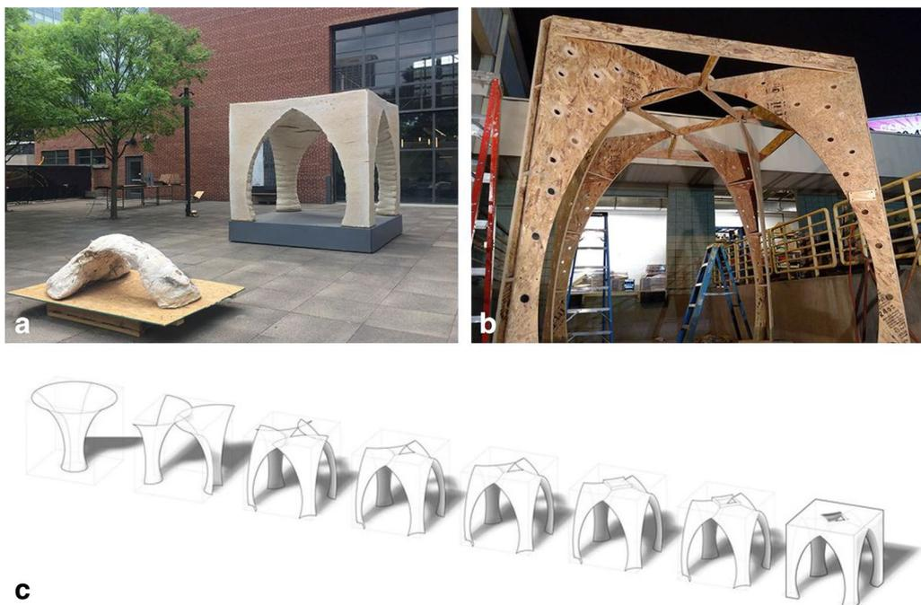
**Fig. 5** a Perspective of the 'El Monolito Micelio' structure and another mycelium composite vault from the "Tactical Mycelium" series [14]. Credit: © Jonathan Dessi-Olive. b The OSB supporting structural skeleton of the pavilion before the combination with the bio-composite. Credit: © Sean Miller. c Diagram showcasing the morphological development of the pavilion [15]. Credit: © Sean Miller
